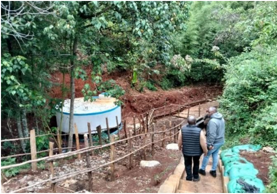
Spring restoration and protection
