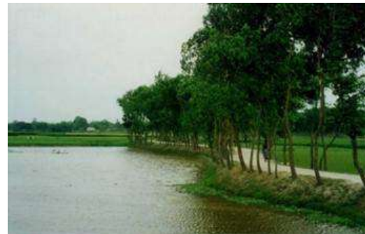
Figure 4.6: Tree Plantation to Protect Embankment/Dykes
